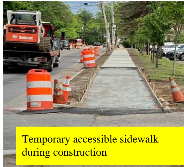
Temp. Asphalt ramp & temp cross walk painted
