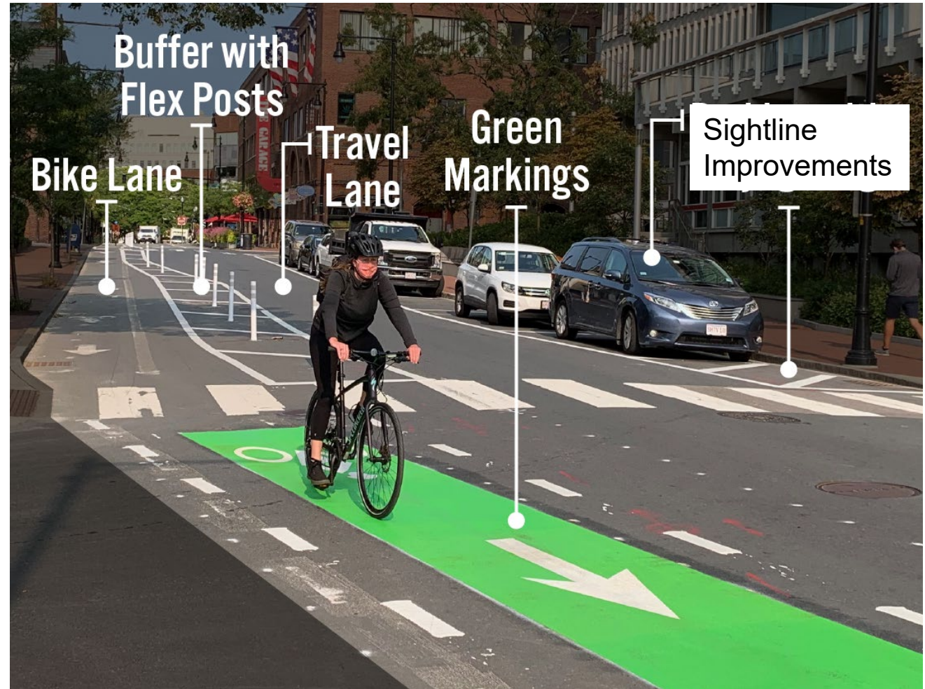
Flexpost and sight line improvement example, Mass Ave Porter Square Safety Improvement Project, Cambridge, MA
