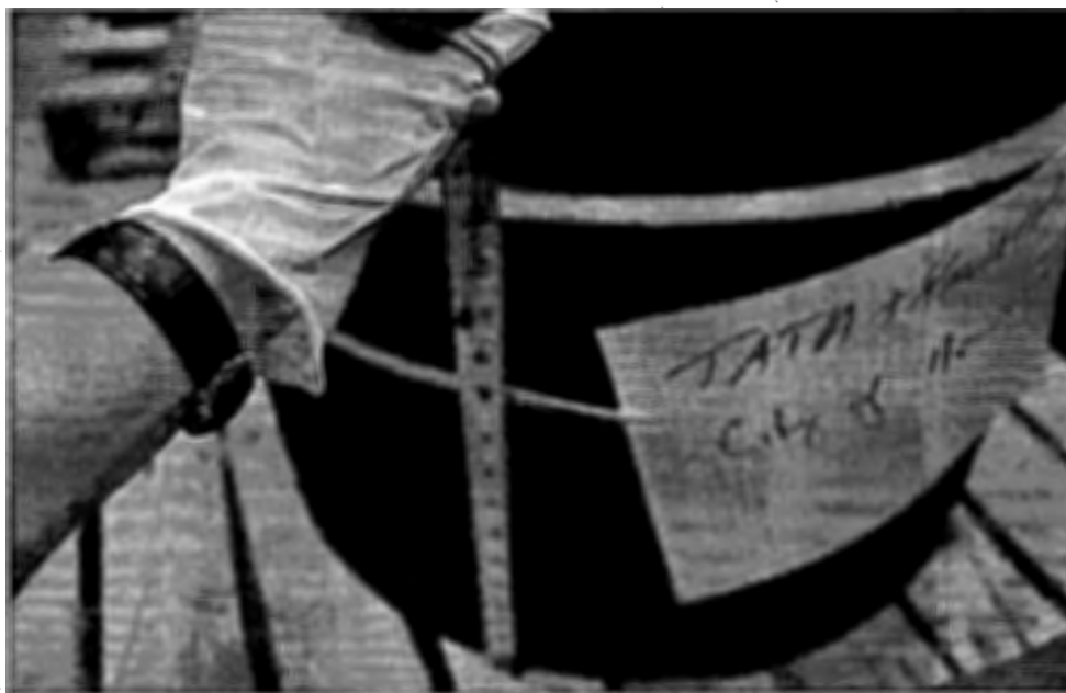
Figure 4: An overall view of a region of wall with corrosion from both ID and OD.
