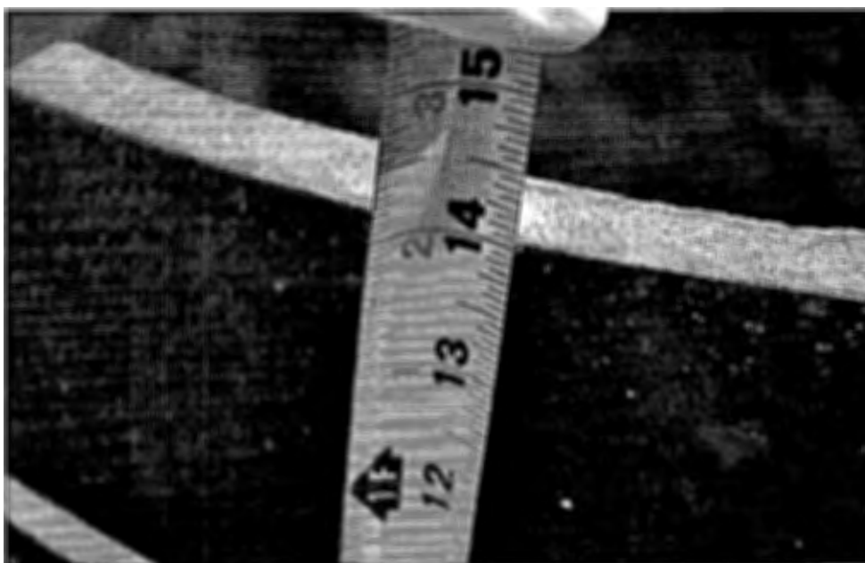
Figure 2: The pipe segment was 14-inches long.
