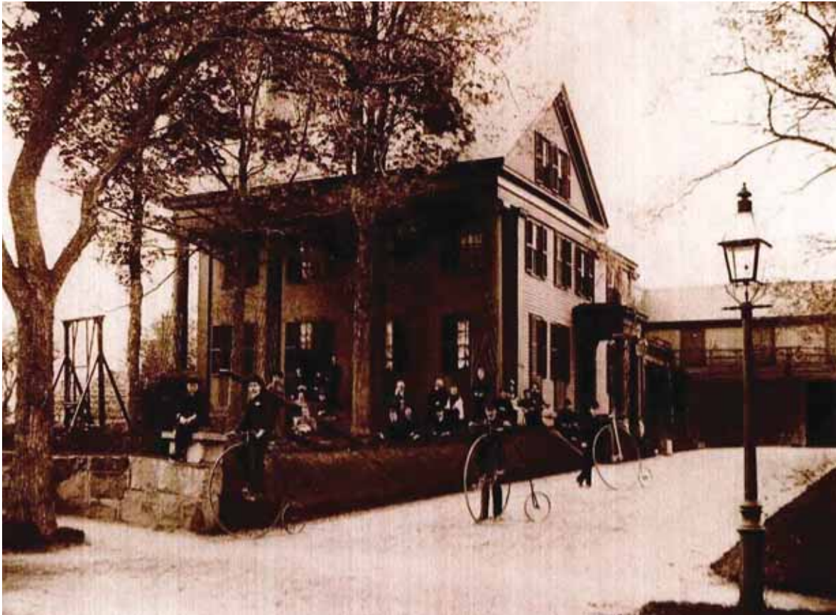
Nathaniel Allen House, Description of Rehabilitation
