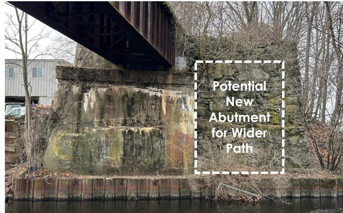
Existing South Substructure
