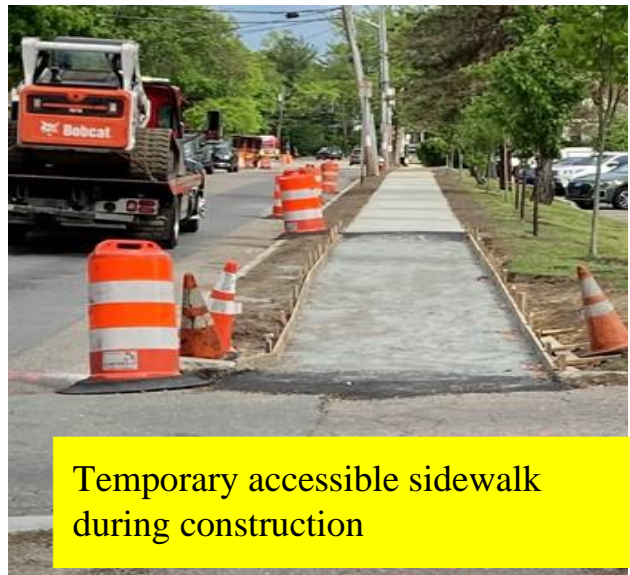
Temp. Asphalt ramp & temp cross walk painted
