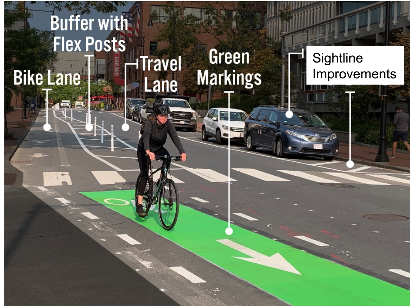
Flexpost and sight line improvement example, Mass Ave Porter Square Safety Improvement Project, Cambridge, MA
