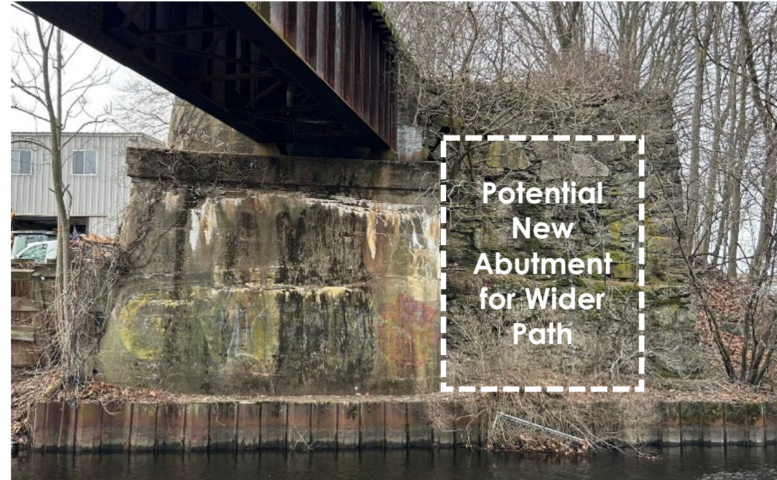
Existing South Substructure
