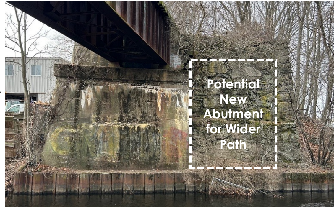
Existing South Substructure
